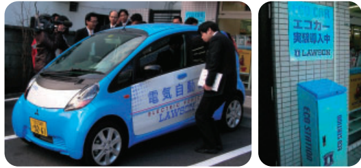
Lawson installed a 200V battery charging station at a test store in Tokyo's Koto Ward.
